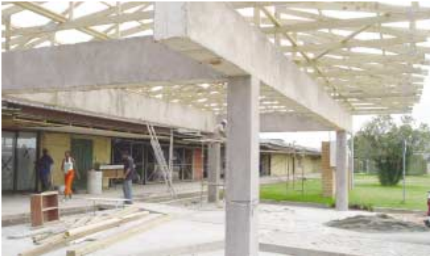
Alterations to Cecilia Makiwane Hospital in Mdantsane outside East London.
